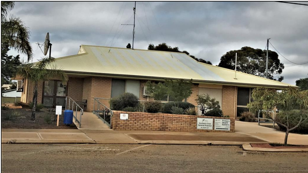
IMAGE: SOUTHERN CROSS GENERAL PRACTICE – ACCESSIBLE RAMP AND HANDRAILS
